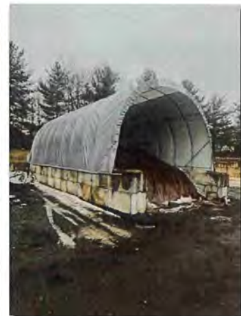
Repaired salt tent
