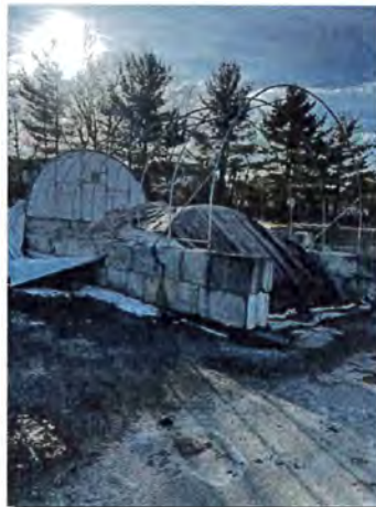
Wind damage to salt tent
