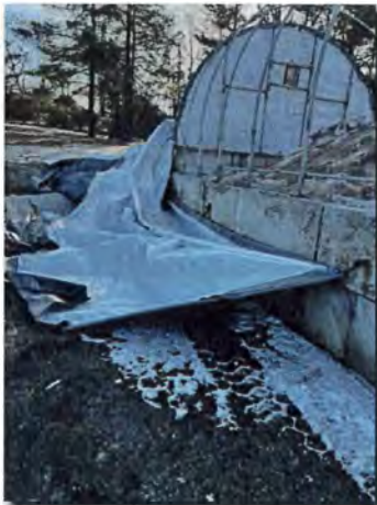
Wind damage to salt tent
