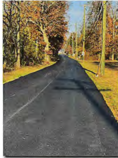
Barclay Rd. Scratched and Paved
