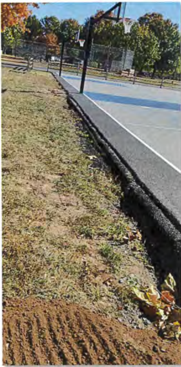
Initial Edge / Dropoff After Paving
