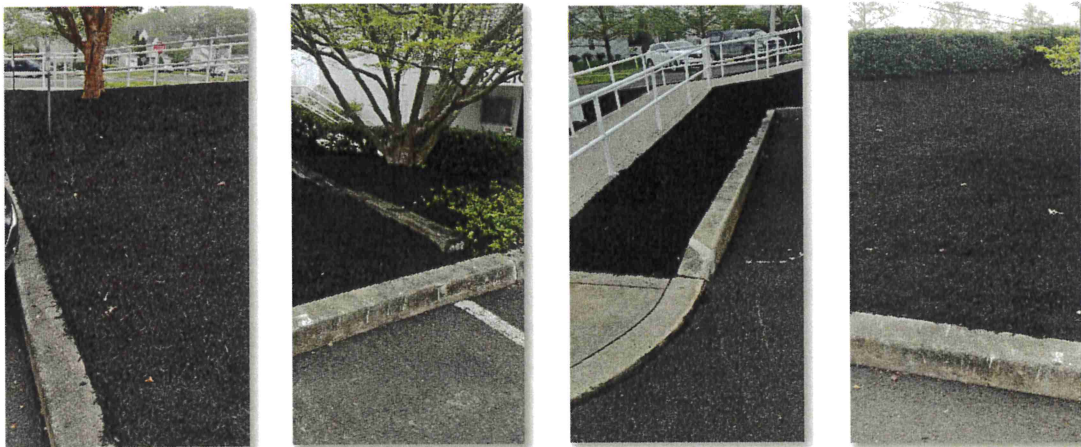
All Above Pictures are of the Finished Area by the Police Entrance
