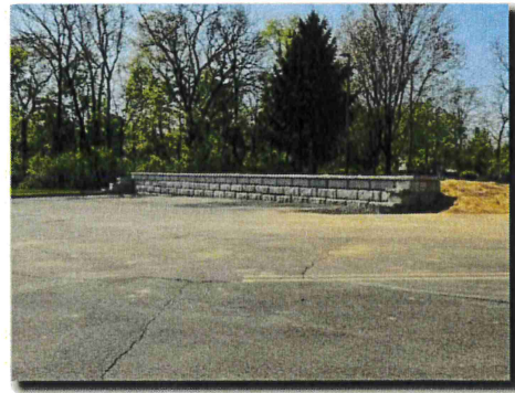
New Block Retaining Wall
