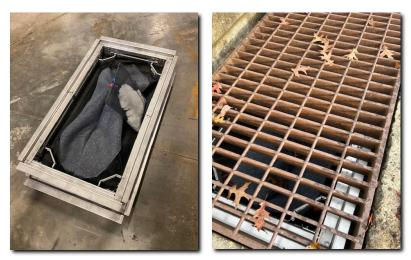
Flexstorm Inlet Bags before and after installation.
