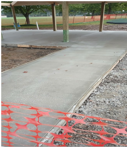
Poured Concrete access off Main Drive
