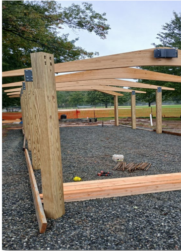
Posts set and Rafters installed
