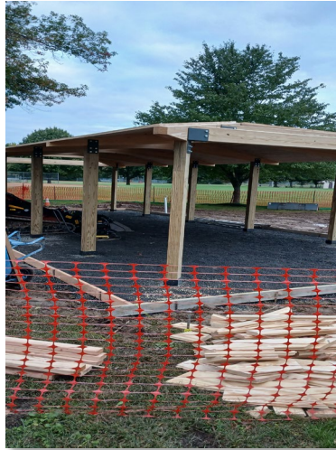
Roof Timber Installed
