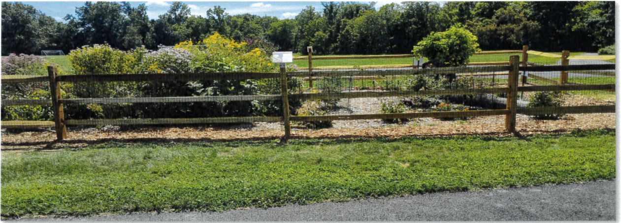
Above picture shows completed project with information signs installed
