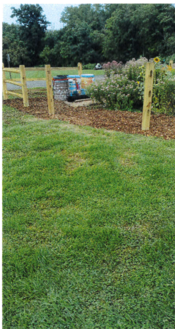
Finished Expansion w/ Posts Installed
