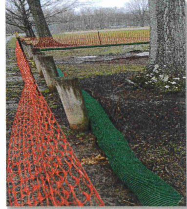
Silt Sock Installation
