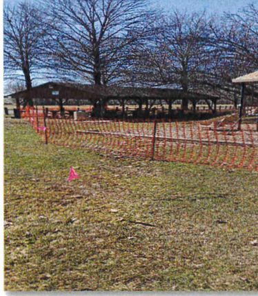
Safety Fence Installation
