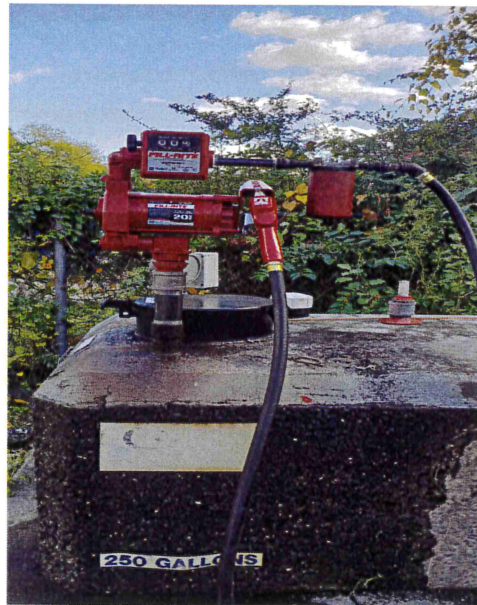
New Pump After Installation
