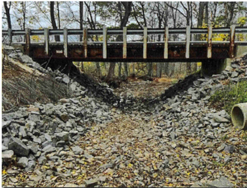
Keller Rd. Bridge Streambank Restoration
