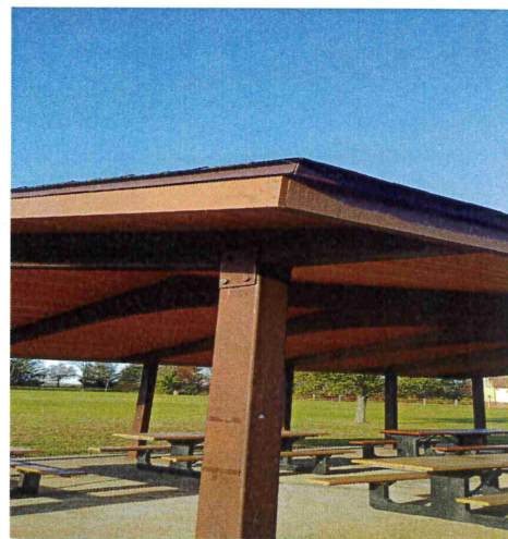
New Fascia Installed and Painted
