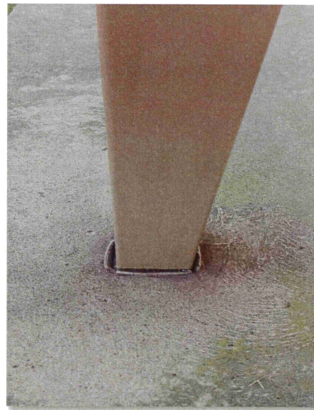
Finished Painted Post
