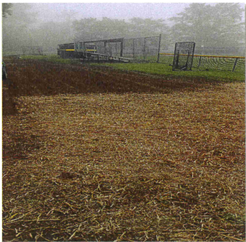
Graded Topsoil with Seed and Straw
