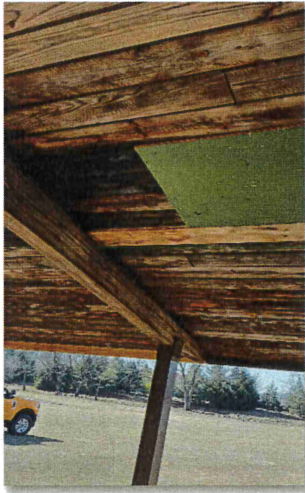
Wood Rotting Past Patched Area
