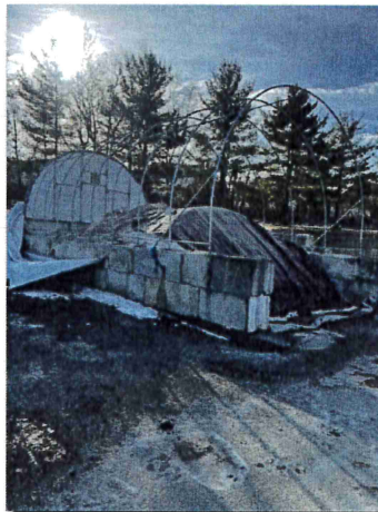
Wind damage to salt tent
