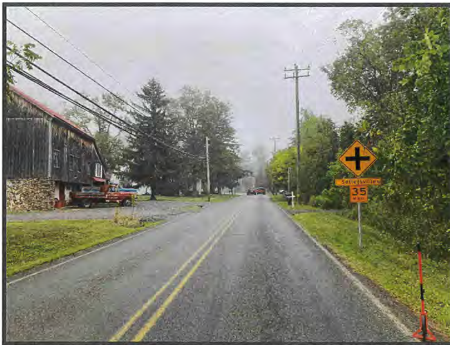
Figure 2: Northbound New Galena Road Approach
