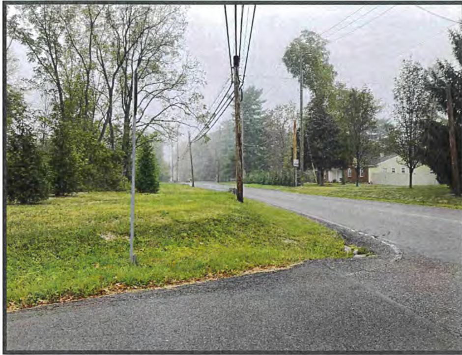
Figure 6: EB Sellersville Road Looking Left
