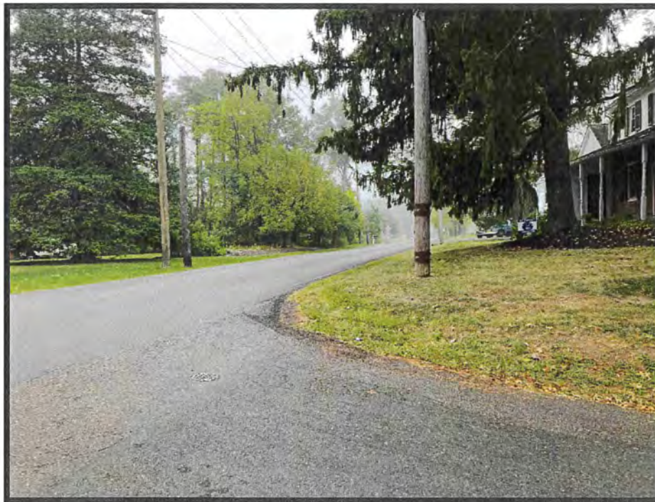
Figure 7: EB Sellersville Road Looking Right
