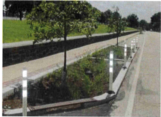
Figure 8. Traffic Bump Out - City of Philadelphia
