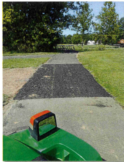
Fresh Asphalt Patch
