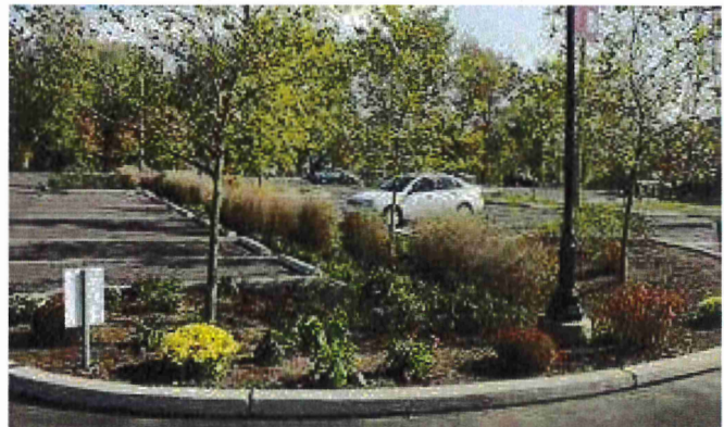
Figure 1. Shade trees planted in rain garden with shrubs and perennials to enhance growing conditions Montgomery County Community College West Campus, Pottstown Borough
