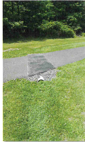
Completed project with blacktop.
