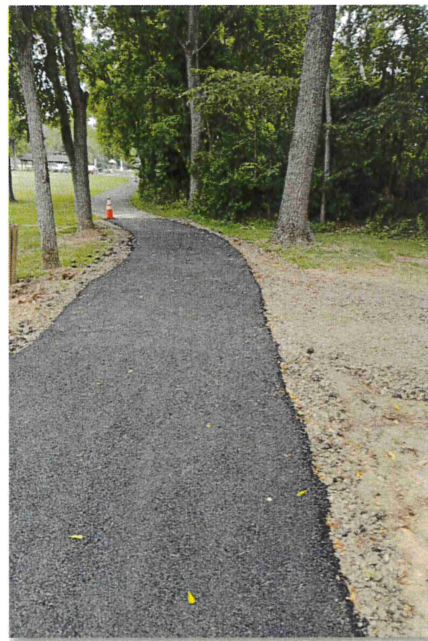
Fresh Asphalt Compacted
