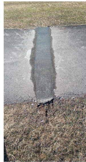
Saw cut around entire crack Debris Removed and Stone Compacted Filled with Concrete
