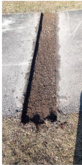
Saw cut around entire crack Debris Removed and Stone Compacted Filled with Concrete
