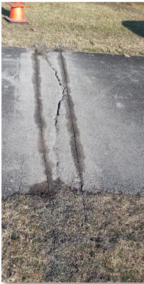
Saw cut around entire crack Debris Removed and Stone Compacted Filled with Concrete
