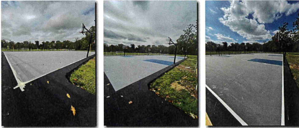
Stages of the sealing and striping of basketball courts at North Branch Park
