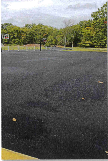
Bare court prior to application
