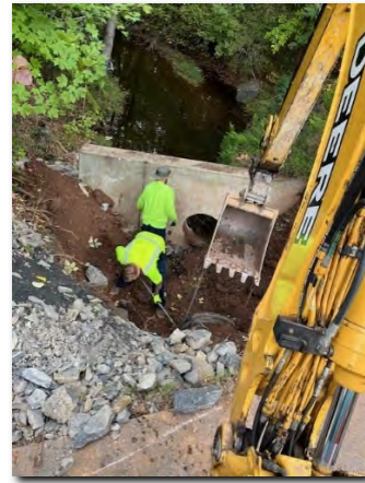
Skyline Drive Culvert before and during repairs.
