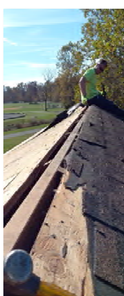
Removal of shingles and ridge cap
