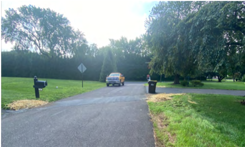
#3 Clearview Ave. completed pipe repairs.
