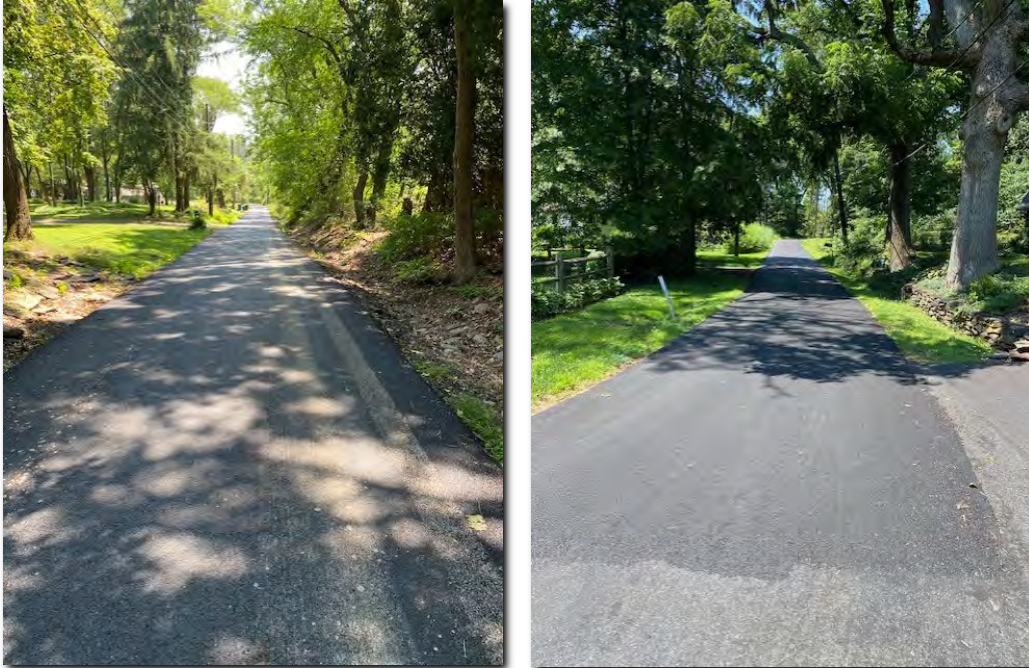
Chapman rd. scratch/ leveling.
