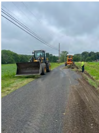
King Rd. re-graded ditch line.
