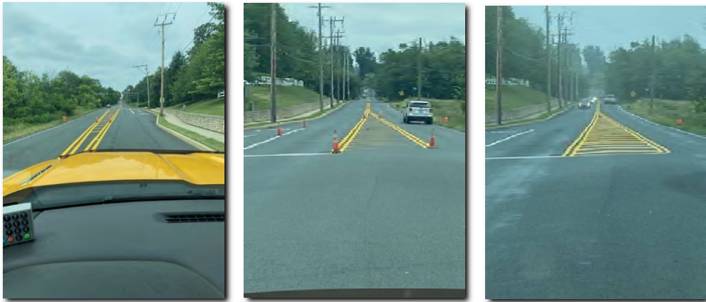
Upper State Rd. Line Striping.
