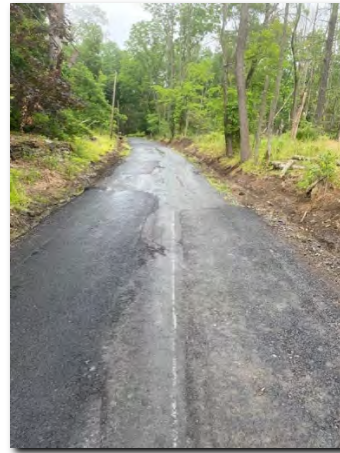
Chapman Rd. re-graded ditch lines.
