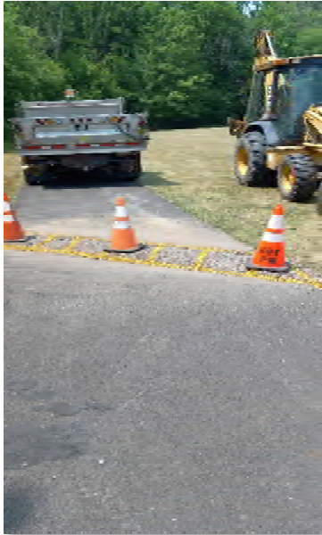
Pipe installed with compacted stone.
