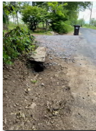
Chapman Rd. Driveway Pipe
