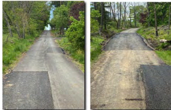
Chapman Rd. base repairs
