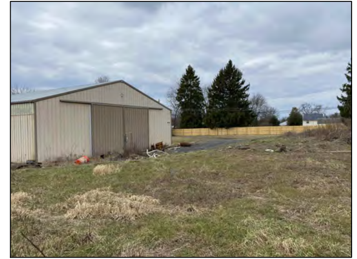
16 VIEW OF EXISTING GARAGE
