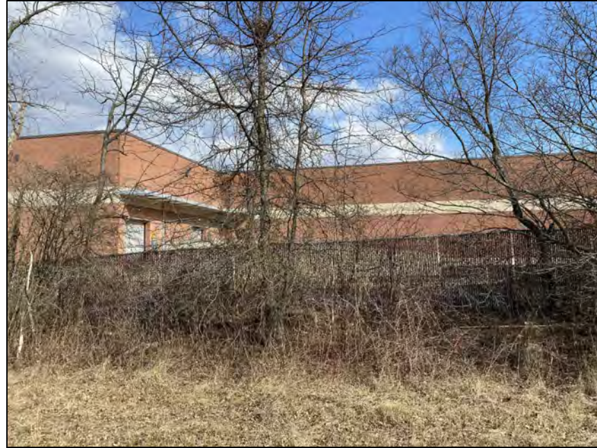
9 VIEW OF EXISTING ADJACENT BUFFER TO EXTRA SPACE STORAGE
