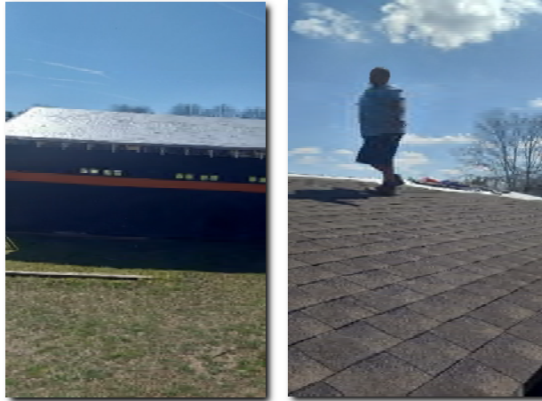
Before and after shingles on dugout Roof.
