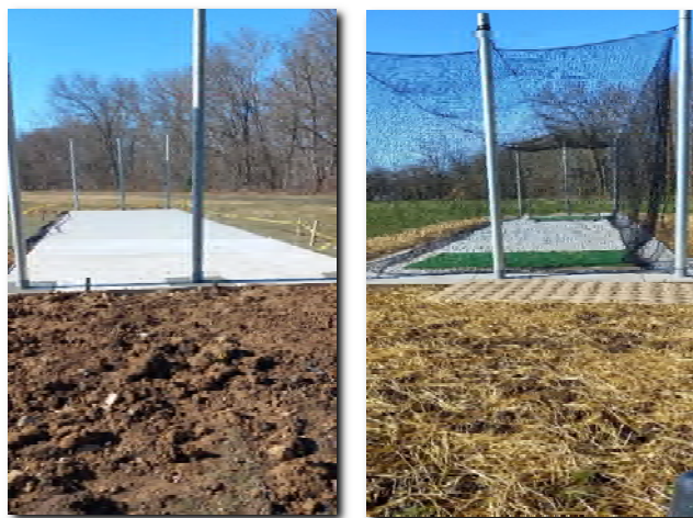
During and after construction of batting cage on Field #4.
