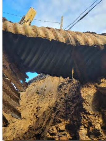
Walter Rd. Deteriorated Pipe
