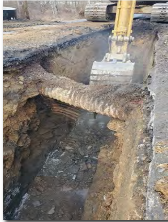
Walter Rd. Deteriorated Pipe
