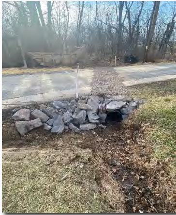
Walter Rd. Completed Pipe Replacement
