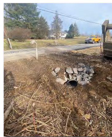
Walter Rd. Completed Pipe Replacement
