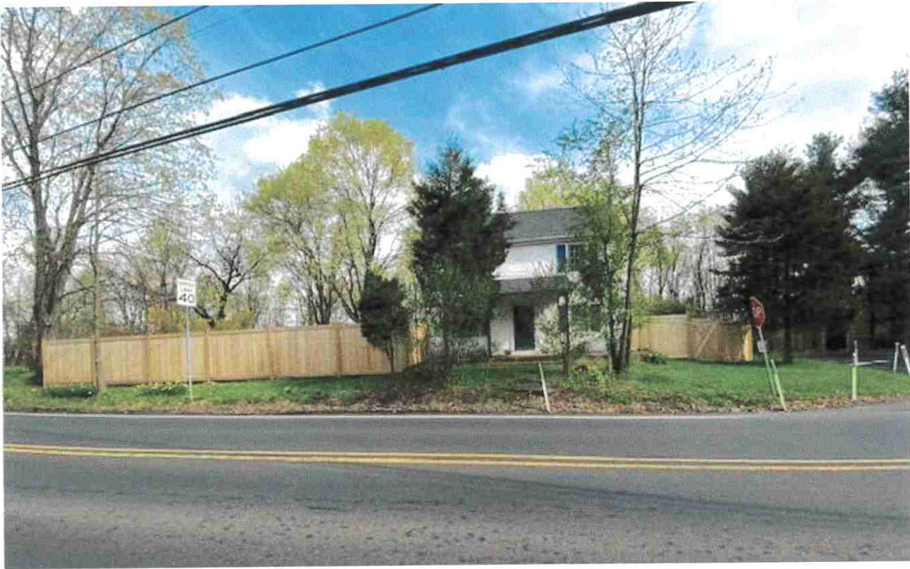
View from Park Avenue/Callowhill Road
