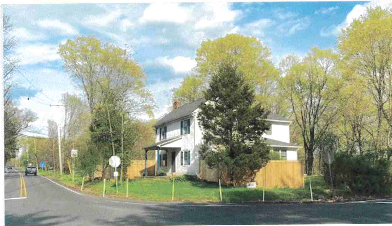
View of fence located between house and driveway
